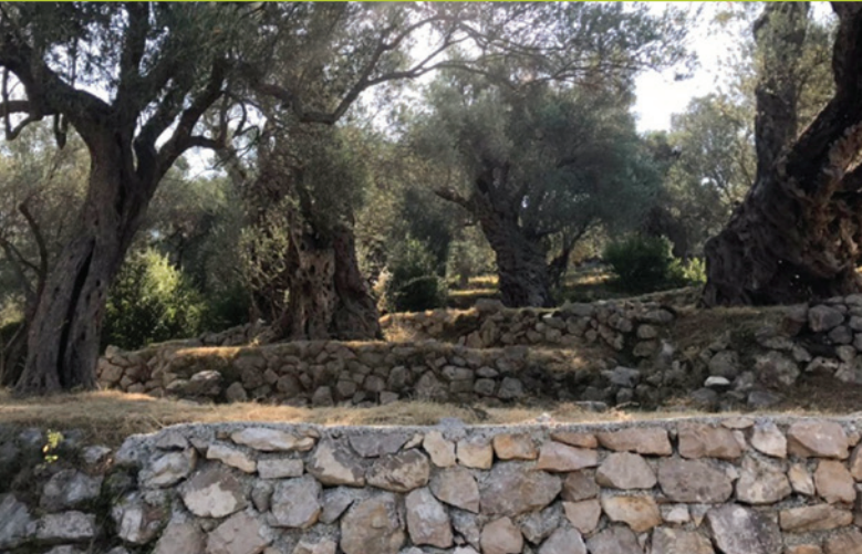
Photo 15. Terracing as an ancient anti-erosion measure
